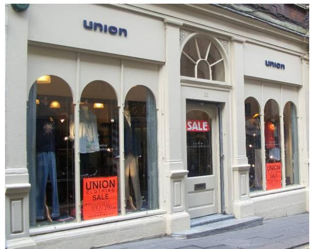
The pilasters above clearly define the entrance and the outer limits of the shopfront, and feature a moulded plinth at the base.
