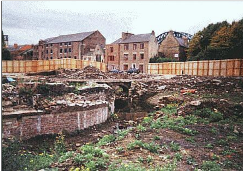
Pandon Burn Culvert, uncovered during construction works, Broad Chare
