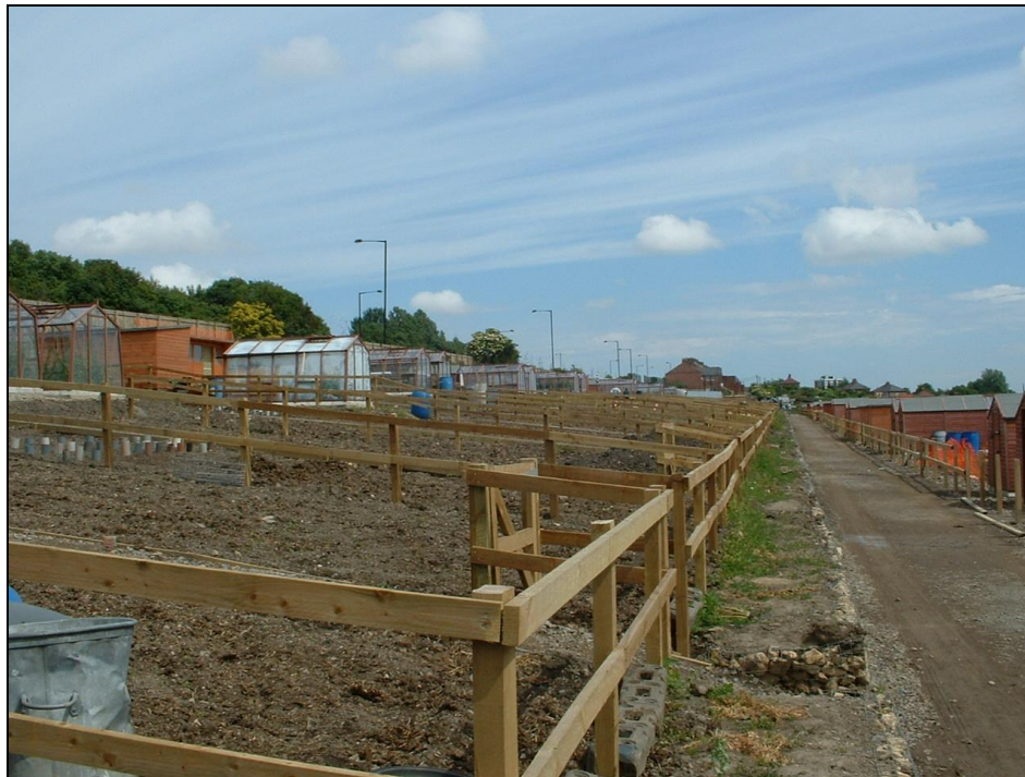
Walker Road Allotments following completion of the site remediation.
