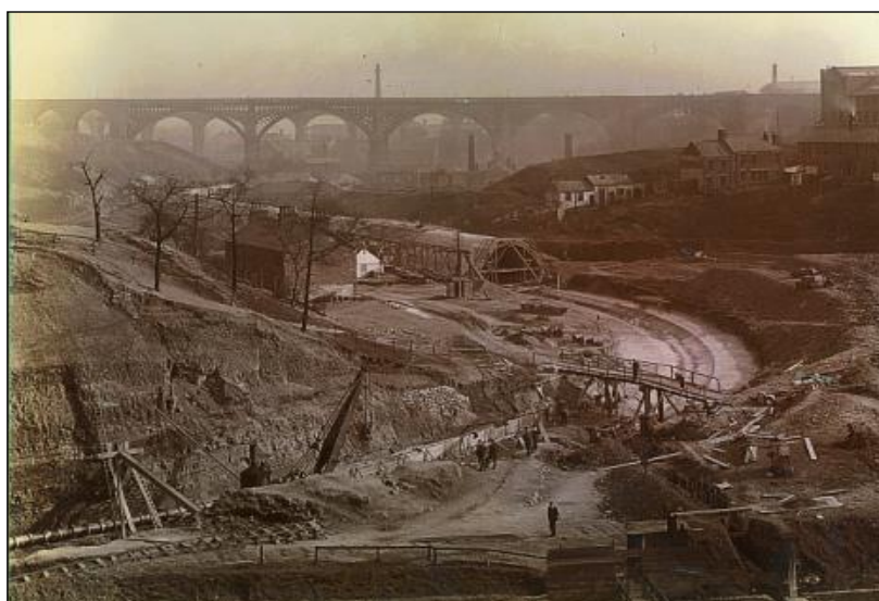
The Construction of the Ouseburn Culvert 1907
